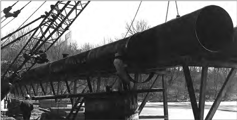
■ Corrugated steel pipe aerial sewer.
