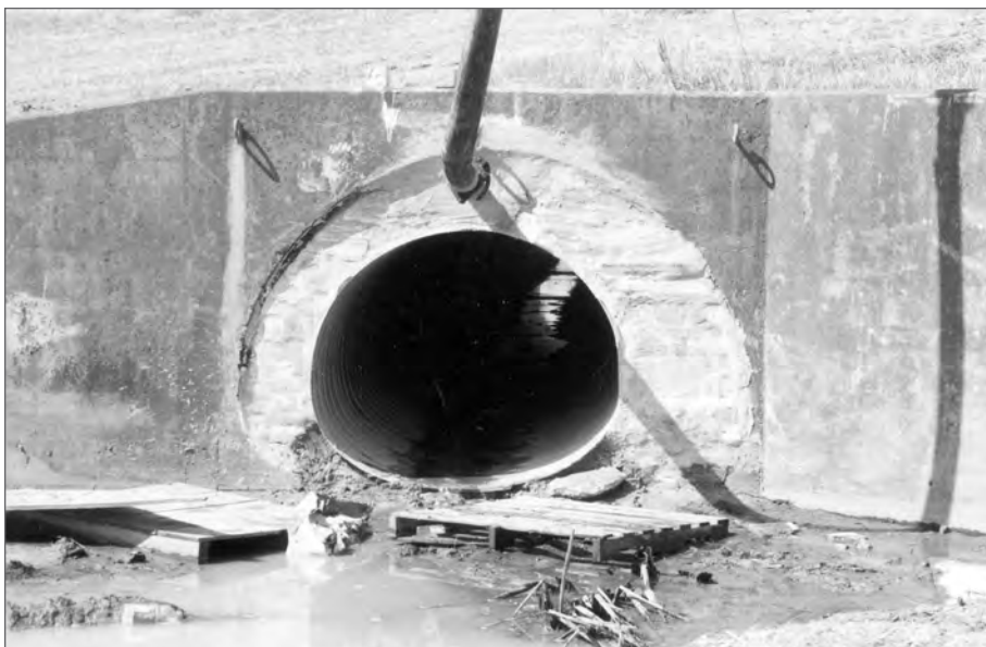
■ Figure 12.14 Grout can be pumped into annular space through an opening in the end bulkheads.
