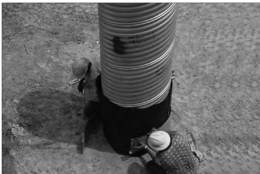
■ Figure 10.16 CSP manhole being installed.
