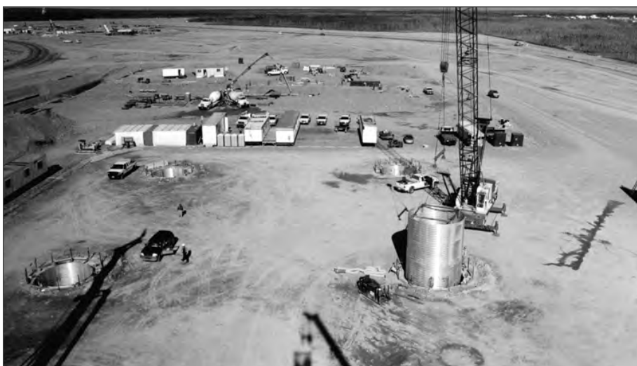
■ Inserting the structural plate shaft liner.
