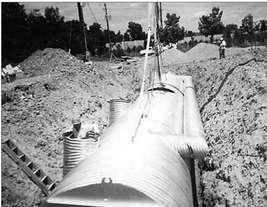
■ CSP sand filter system
