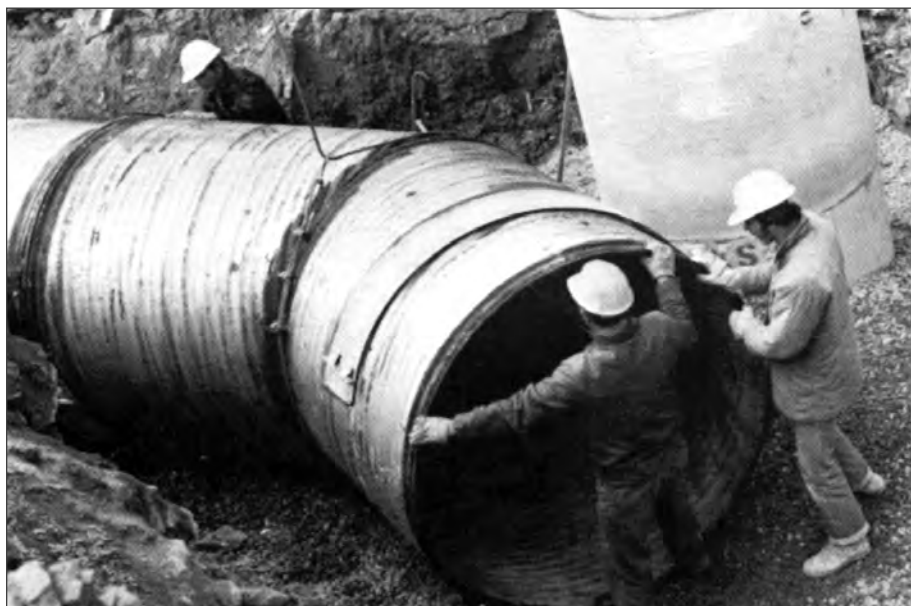
■ Figure 10.14 Pre-fabricated miter section of CSP is lowered into place to match bend in trench.
