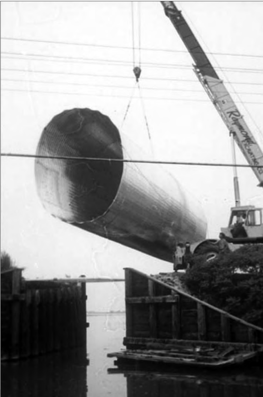
■ Figure 10.44 Assembled structure being placed in position.
