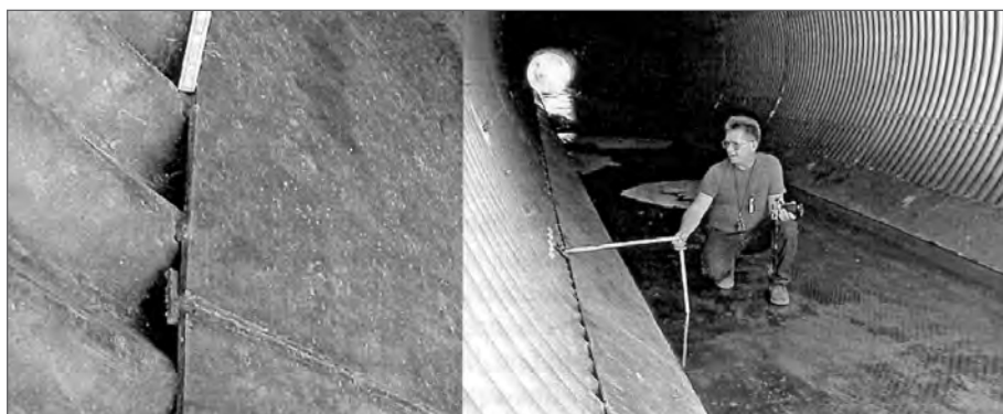
■ Figure 12.16 Steel armor-plated invert.
