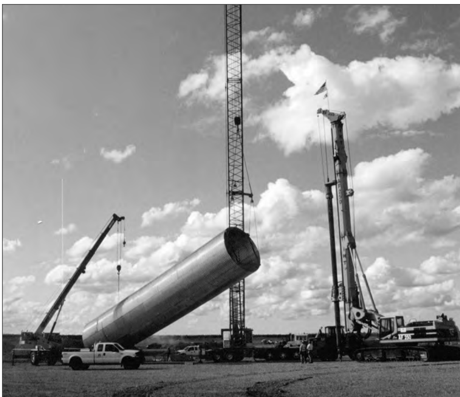
■ A 16 foot diameter structural plate shaft liner is picked up to be inserted in a bored shaft.
