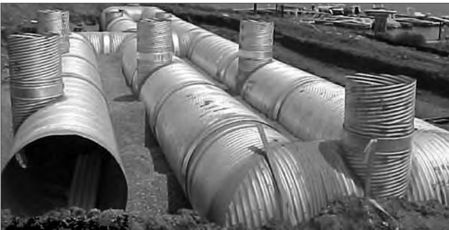
■ CSP riser manholes in underground detention system.
