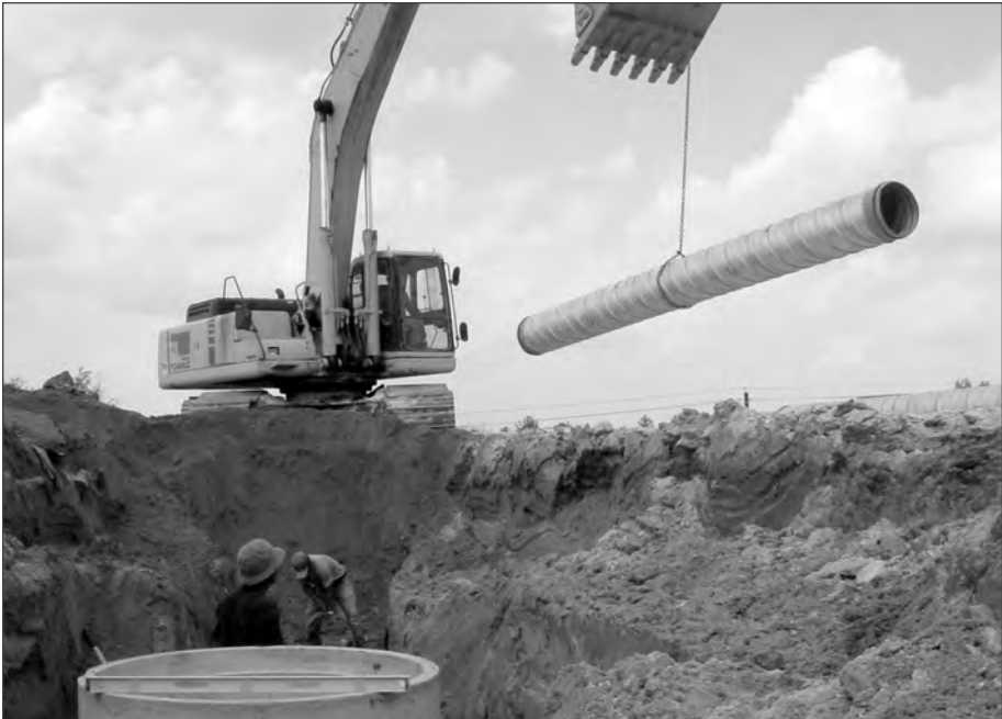
■ Figure 10.12 Lifting CSP into place.
