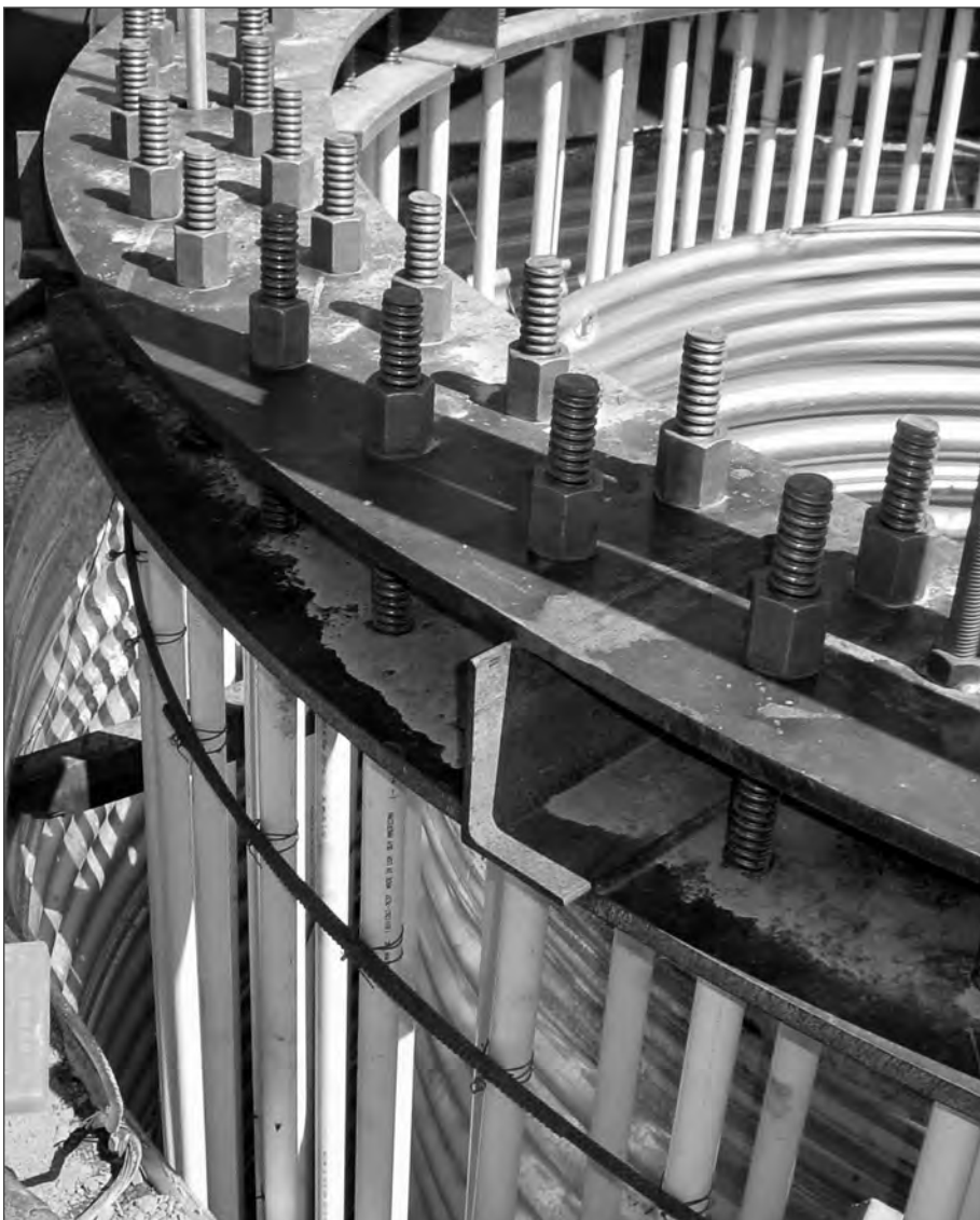
■ CSP form for wind turbine generator footing.
