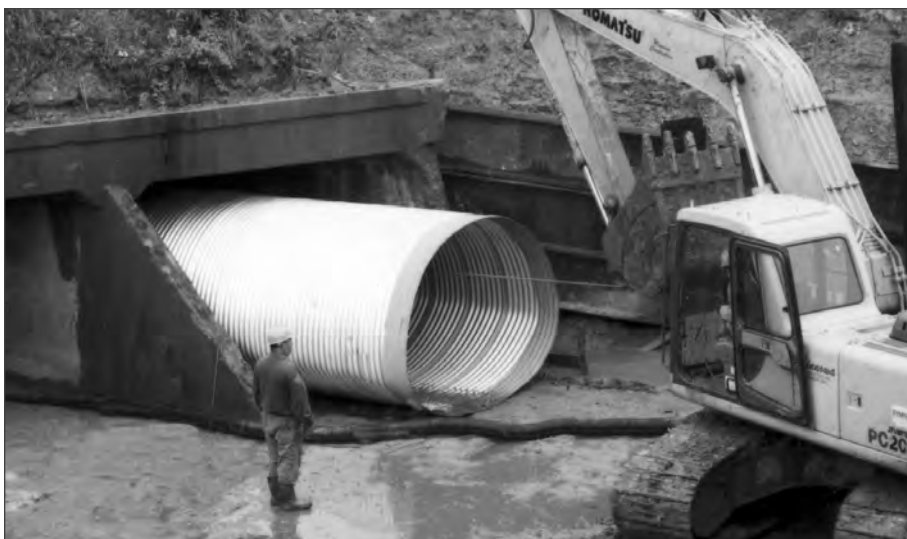
■ Relining of a failed concrete box with corrugated steel pipe arch.
