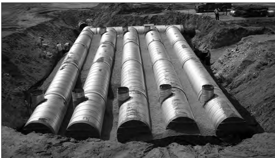
■ CSP underground detention.
