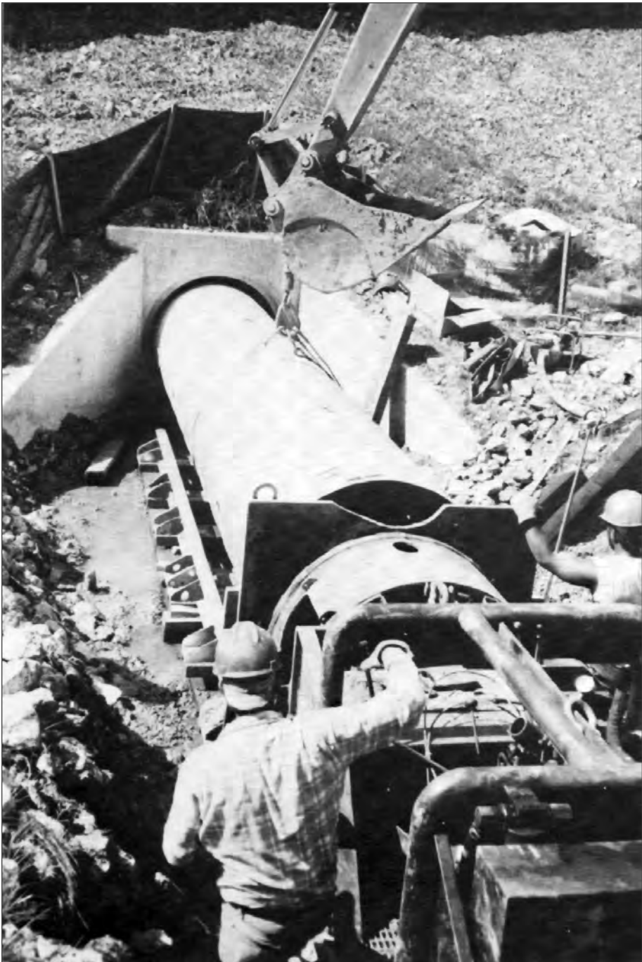
■ Figure 11.1 48 inch diameter CSP being used to slip line failed 54 inch diameter concrete pipe. Class 5, on partially constructed PA DOT Project – Southern Expressway – near the Pittsburgh Airport.
