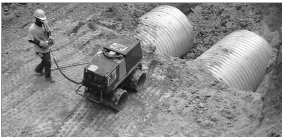
■ Figure 10.1 Proper compaction equipment close to structure.
