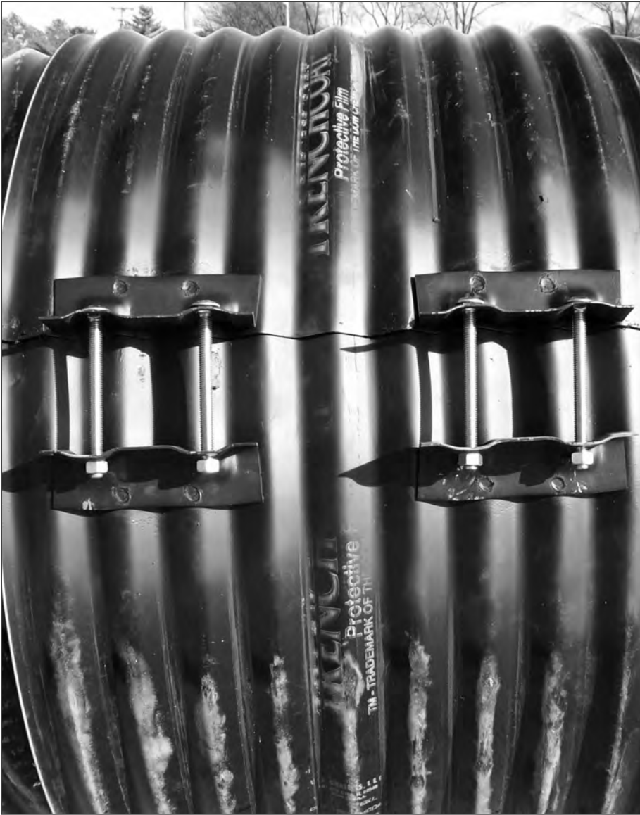
■ Corrugated steel pipe band connectors.
