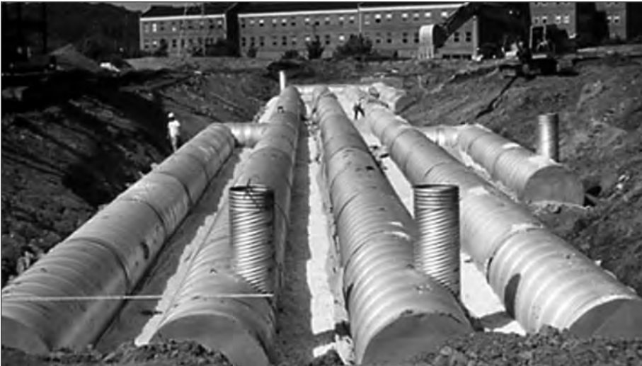
■ Typical CSP underground detention system.
