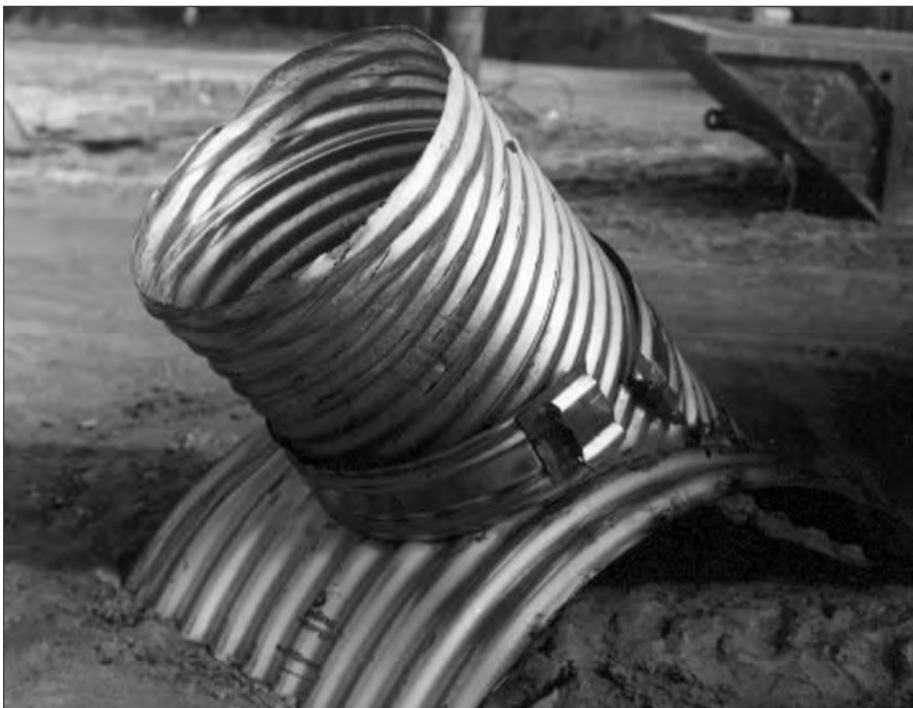
■ Figure 10.18 Typical CSP saddle fitting.
