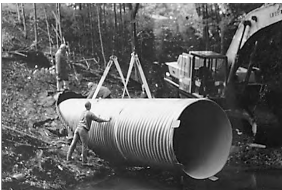
■ Figure 12.19 Slip lining with CSP.
