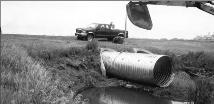
■ Figure 11.5 There are many economical pipe rehabilitation techniques being used. One method employs the use of CSP to slip line distressed reinforced concrete pipe.
