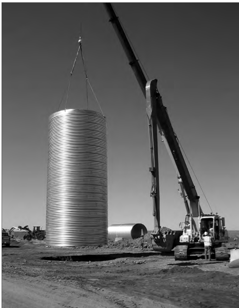
■ CSP form for wind turbine generator footing.
