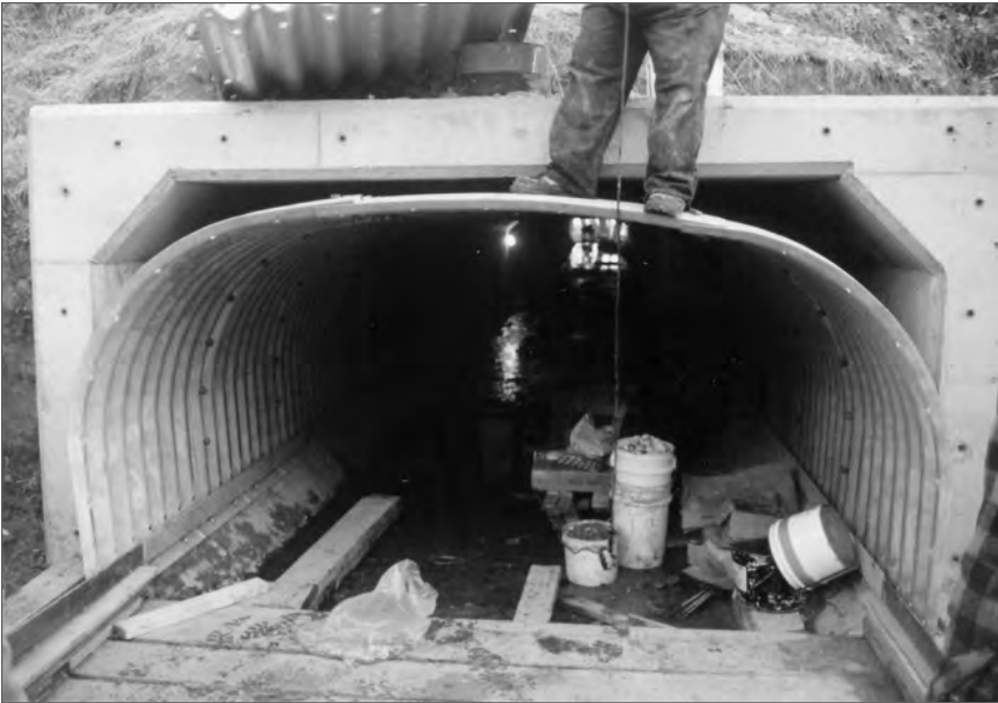
■ Figure 12.12 Lining a concrete box with a steel box culvert.
