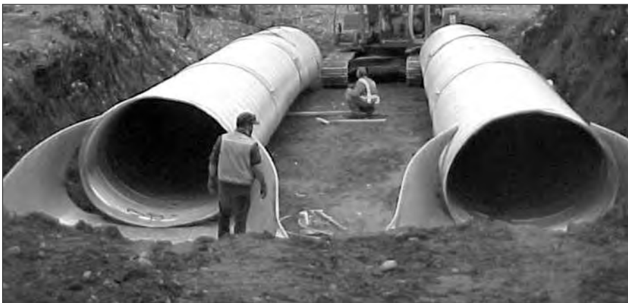
■ Figure 7.24 Pipe arch can be installed in limited headroom situations with shallow cover.
