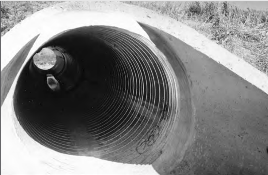
■ Figure 12.15 Finished end treatment.
