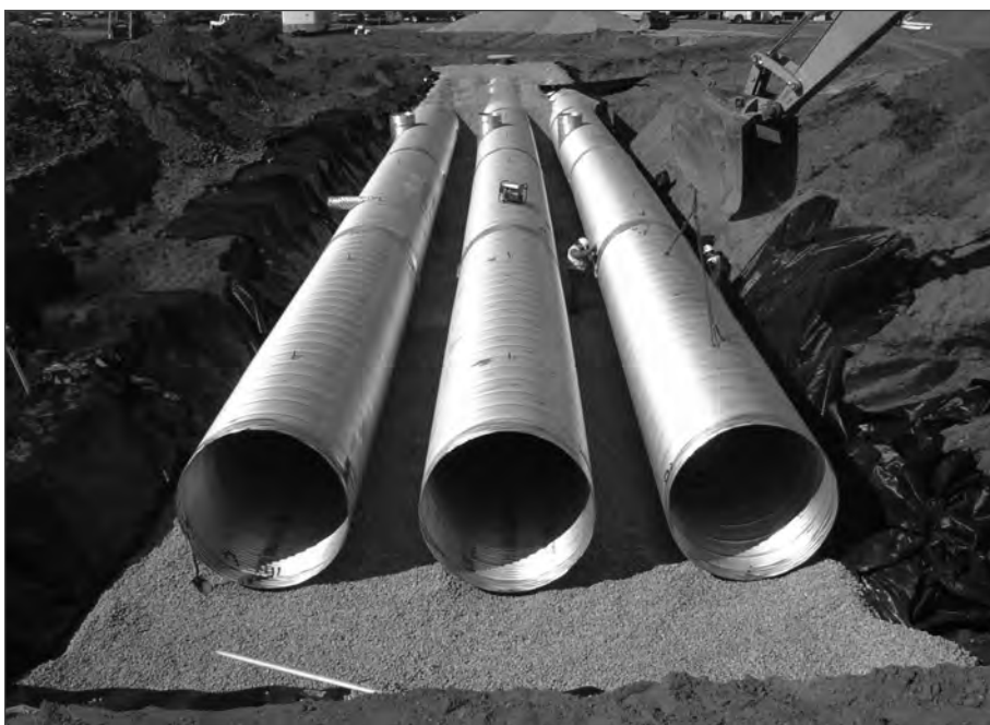
■ Figure 10.33 Detention system installation.
