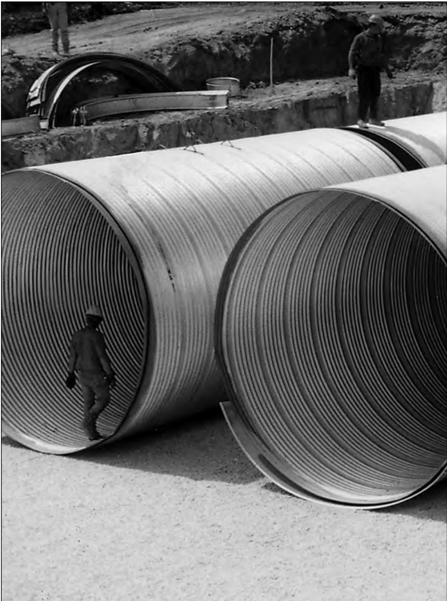
■ Typical CSP underground detention system.
