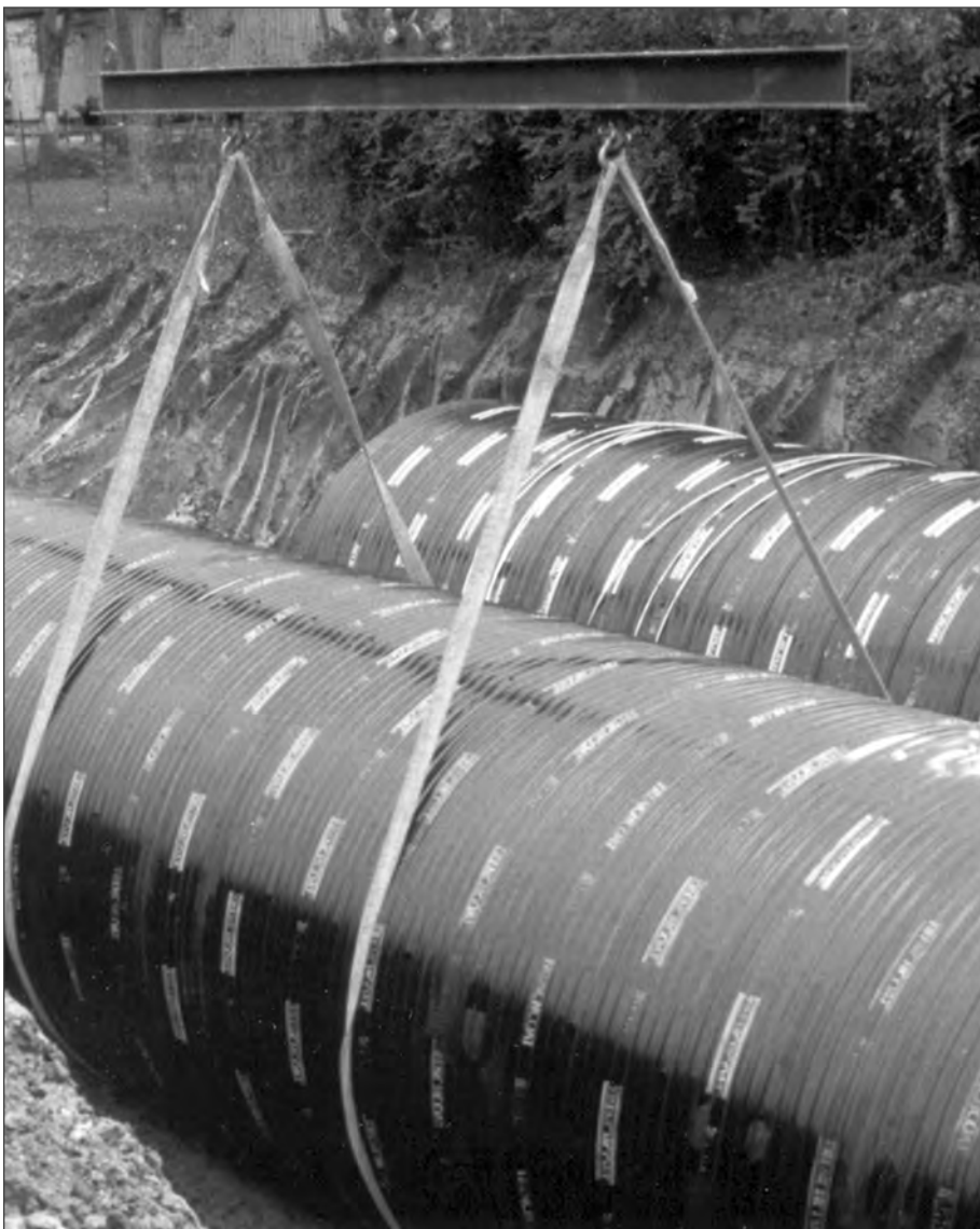
■ Installation of polymer coated CSP.
