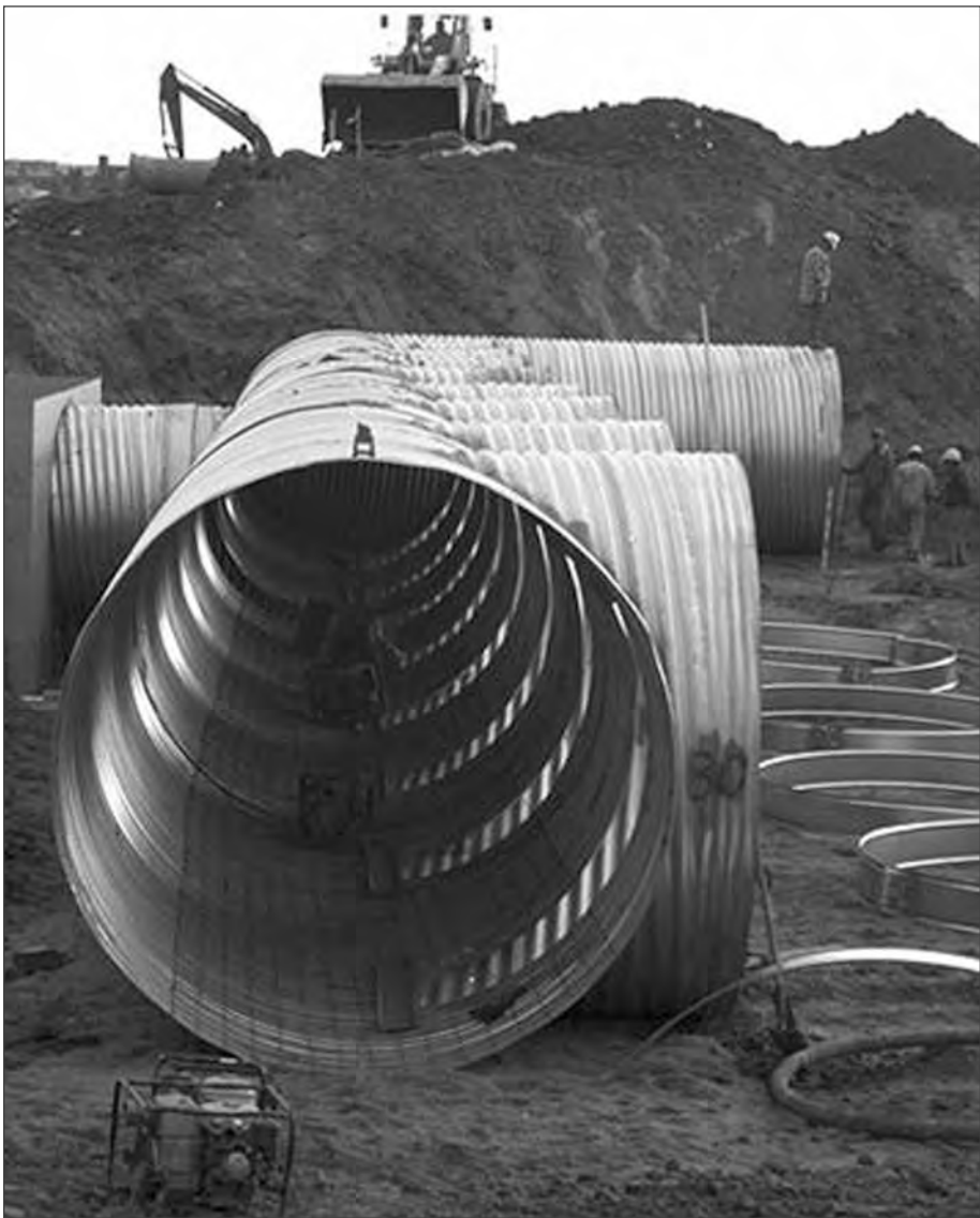
■ CSP underground detention system being installed.
