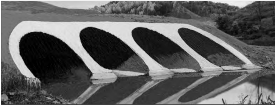
■ Figure 10.31 Multiple line CSP beveled ends.
