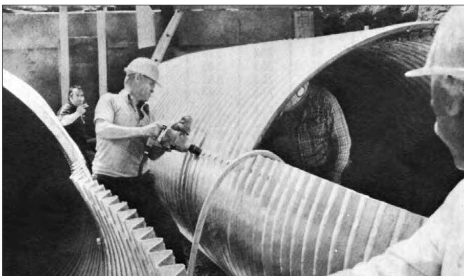
■ Figure 2.9 High-strength steel bolts are used for the circumferential and longitudinal seams of structural plate pipe. Four, six, or eight bolts per foot of longitudinal seam provide the strength required for the loading conditions.
